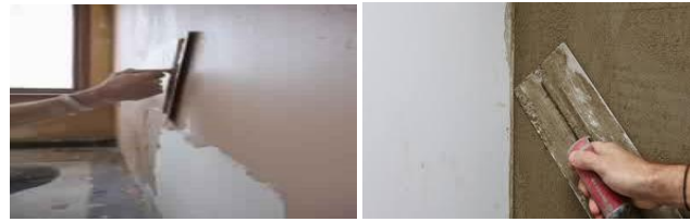
Figure 3.1 a & b are Manual methods of plastering
