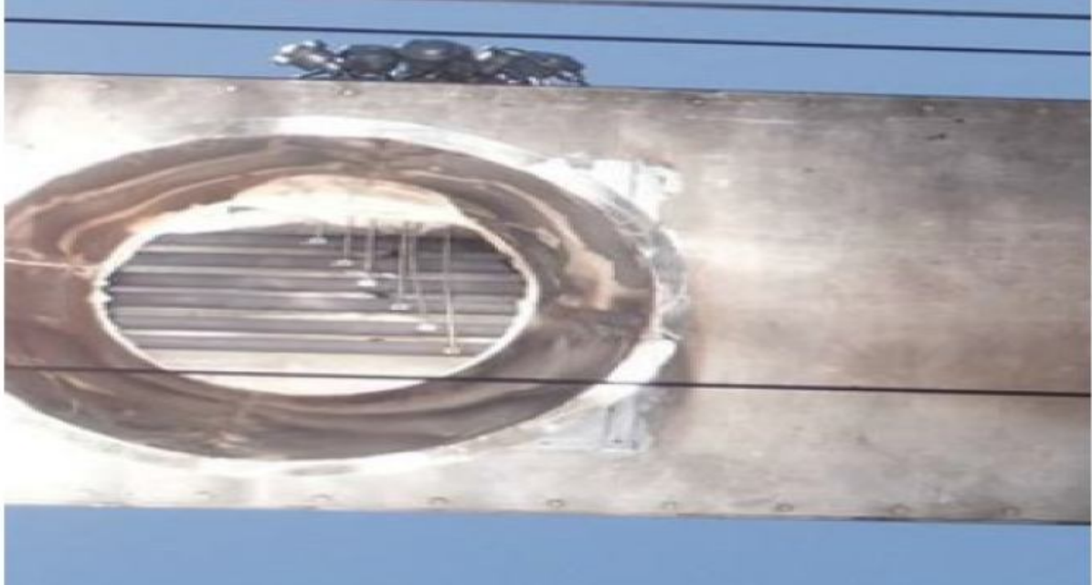
Fig. 7. View on temperature sensors
