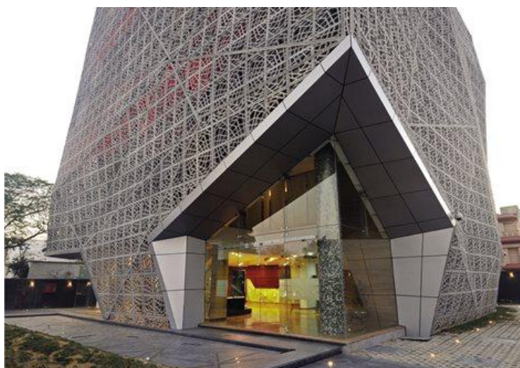
Figure 18:Jali façade, sanjaypuri office, Jaipur
