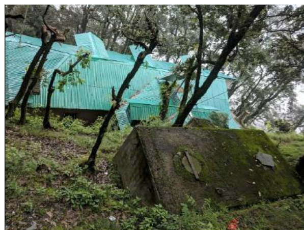
Figure 20. Septic Tank situated in the valleys of Lohali Village (Ward 2)
