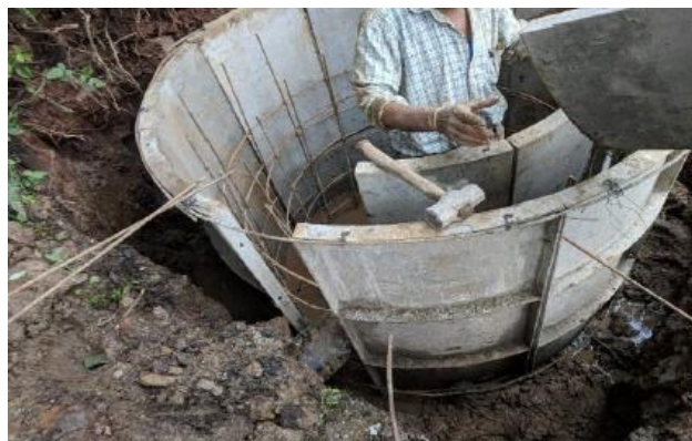
Figure 22. Ongoing construction of septic tank with 2.5m dia and 5m height
