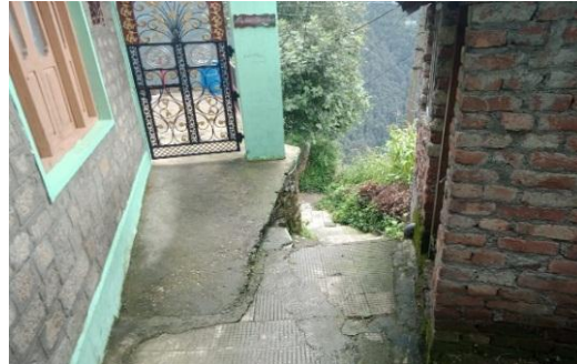
Figure 4. Undulations in terrain in Dalhousie
